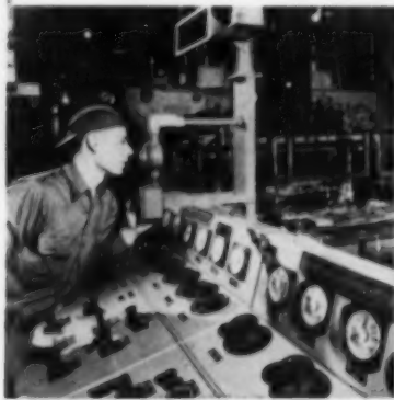
The entire length of the $6,250,000 continuous galvanizing line can be controlled from this panel. Operator keeps in touch with two-way inter-communication set
